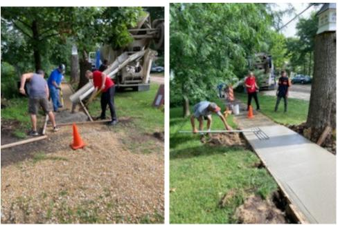
A sidewalk received an update. Old buckled sidewalk was removed and new sidewalk poured. Thanks to Hugh McKiski for lining up the able crew. Hugh and Colton did the forming, Mark and Nick Jensen and Matthew Moore assisted with the pour. Jamie Finnestad did the concrete finishing.
